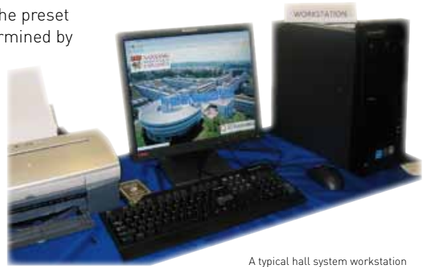
A typical hall system workstation
